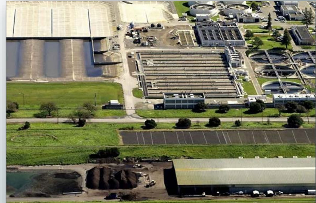
Sewage treated at the Laguna Treatment Plant (LTP) is beneficially reused by the Santa Rosa Regional Water Reuse System
