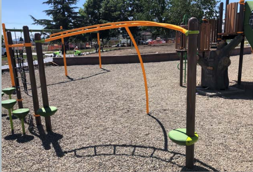
Coffey Neighborhood Park playground construction
