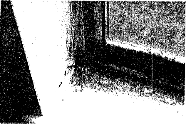
Photo 15 Bedroom 1 - Microbial growth on drywall/sill within window opening
