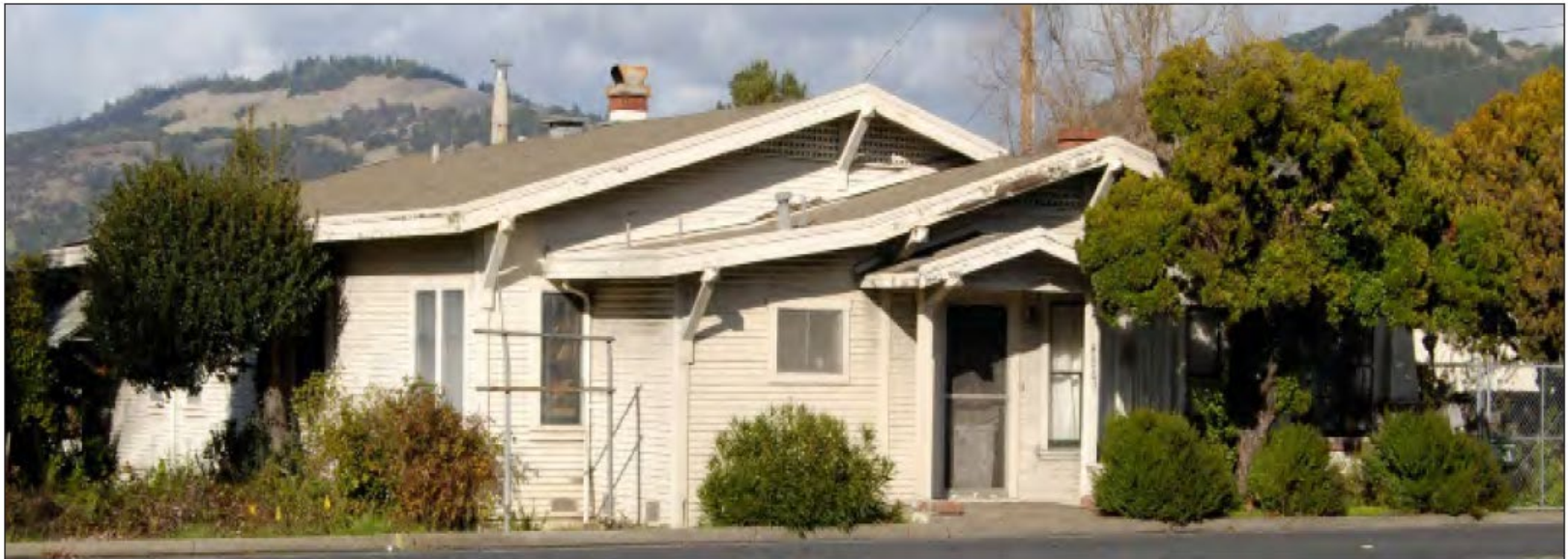
Photo 4. South and west façades, looking northeast across Highway 12 (Sonoma Highway).
