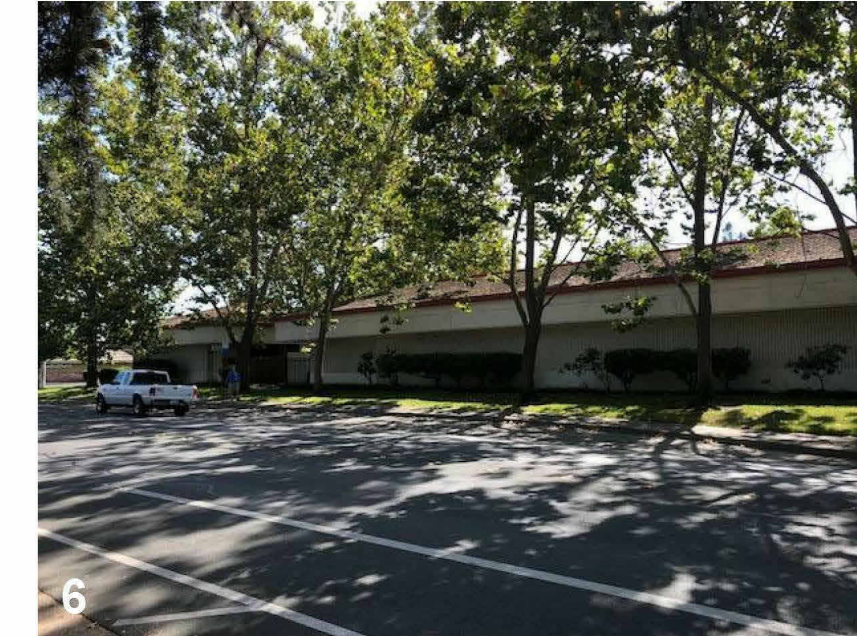
West Steele Lane Elevation of adjacent Retail
