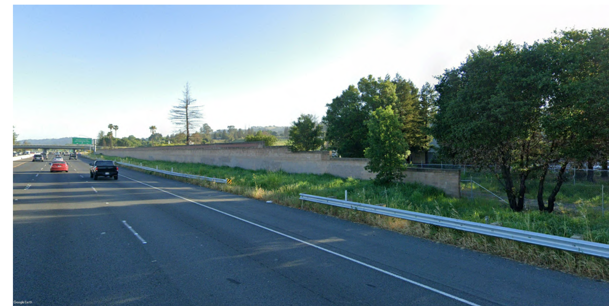
LOOKING FROM HIGHWAY 101 TOWARDS PROJECT SITE ON THE RIGHT
