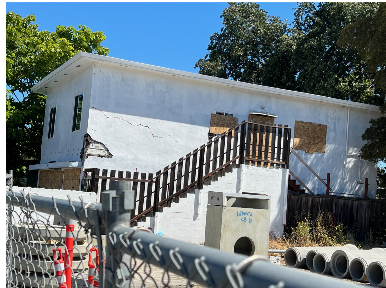
4 VIEW FROM SOUTHWEST STANDING ON S.R. AVE SIDEWALK
