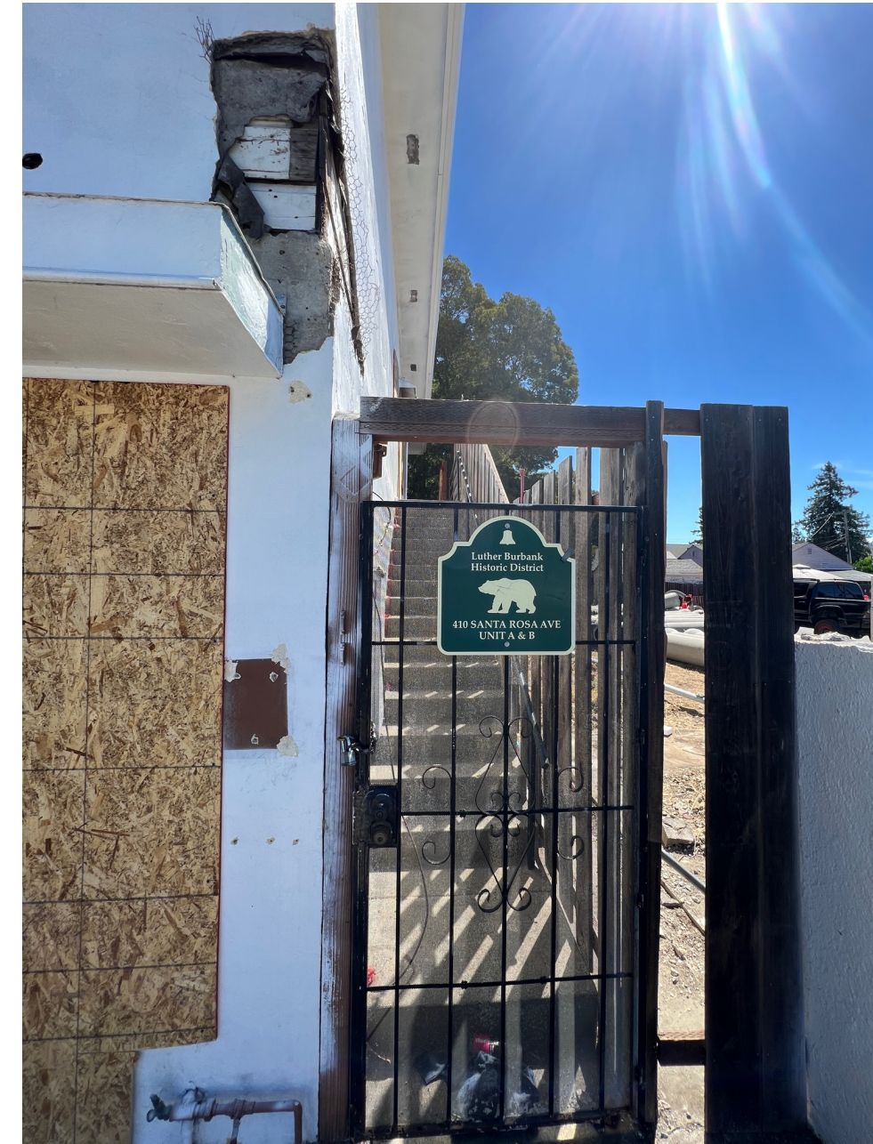
2 VIEW FROM WEST LOOKING UP STAIRWAY
