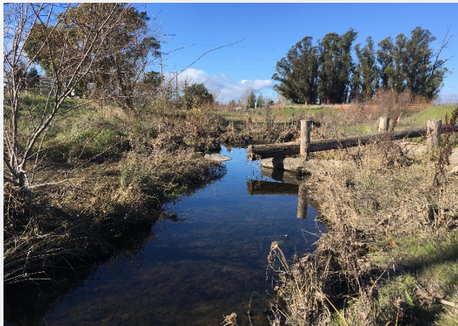
Lower Colgan Creek restoration continued in 2020.
