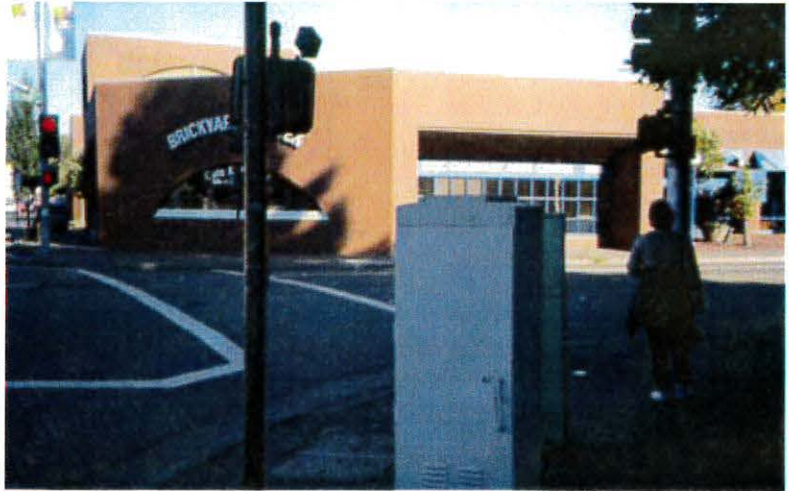
Unightly utility vaults in sidewalk at 7 th and B.
