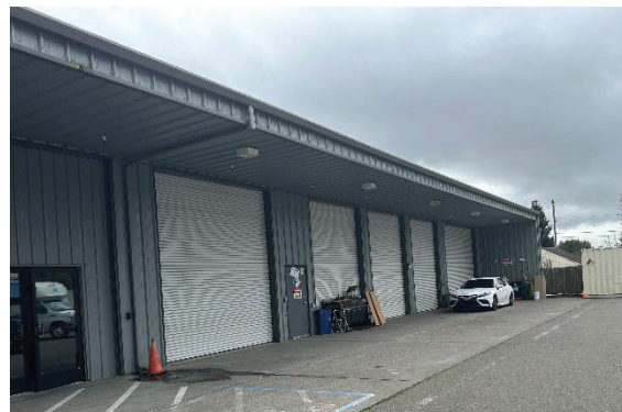
MV's maintenance facility in Santa Rosa
