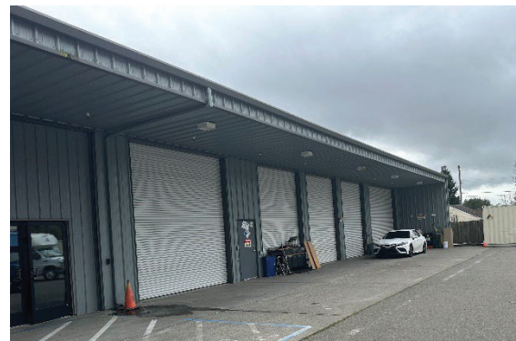
MV's maintenance facility in Santa Rosa
