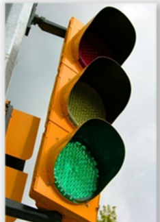
216 Traffic Signals 86 Pedestrian Flashers
