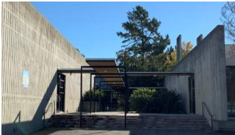
Figure 12: Entry Canopy Between Building 5 and 6
