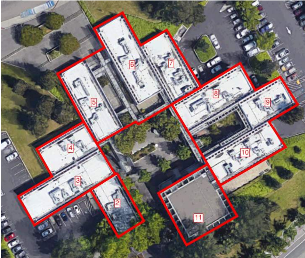
Figure 3: Santa Rosa City Hall - Aerial View
