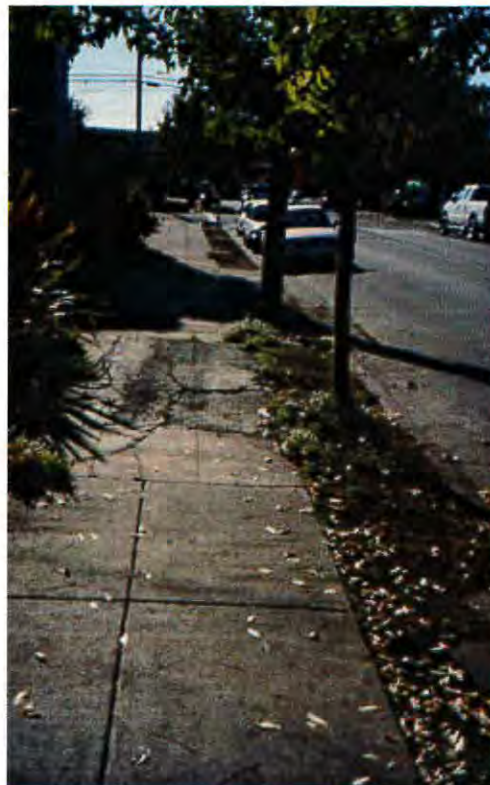
Asphalt patching on a concrete sidewalk on 7 th near Humboldt.
