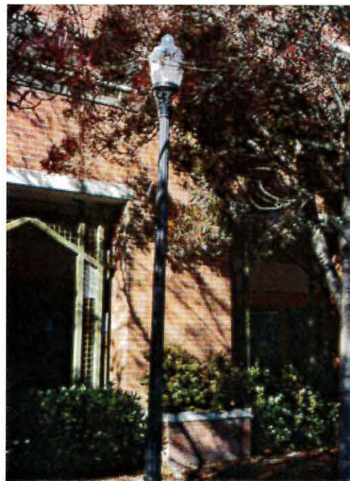
The pedestrian scaled vintage light in front of Parking Garage #7.
