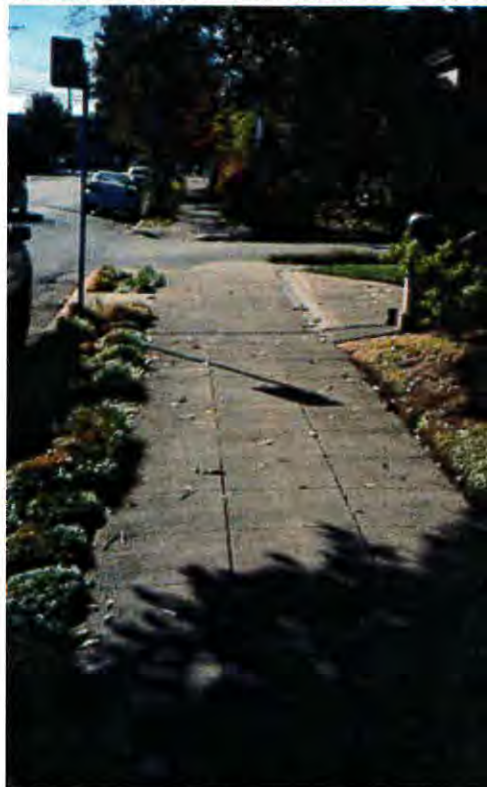
A typical section of historic garden sidewalk on 7 th Street near Orchard Street.
