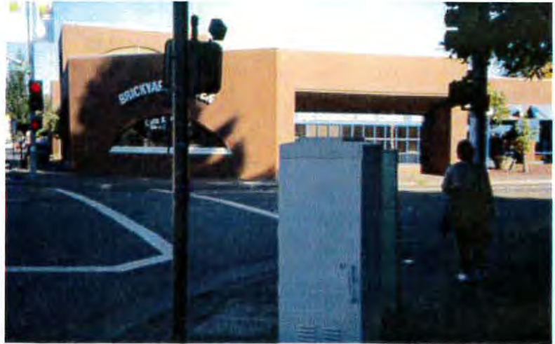
Unightly utility vaults in sidewalk at 7 th and B.
