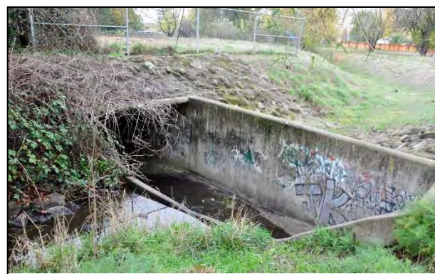
Figure 1: Sierra Park Creek is diverted into the Spring Creek Diversion structure.
