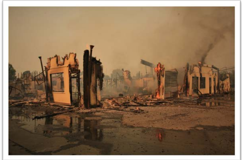
Coffey Park home after its fire was extinguished. Photo by Les Hause, courtesy of John Snetsinger
