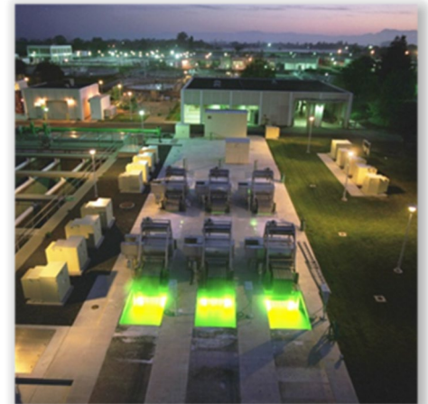
Laguna Treatment Plant
