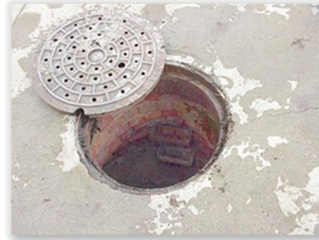
597 Miles of Sewer Mains 12,405 Sewer Manholes 17 Sewer Lift Stations
