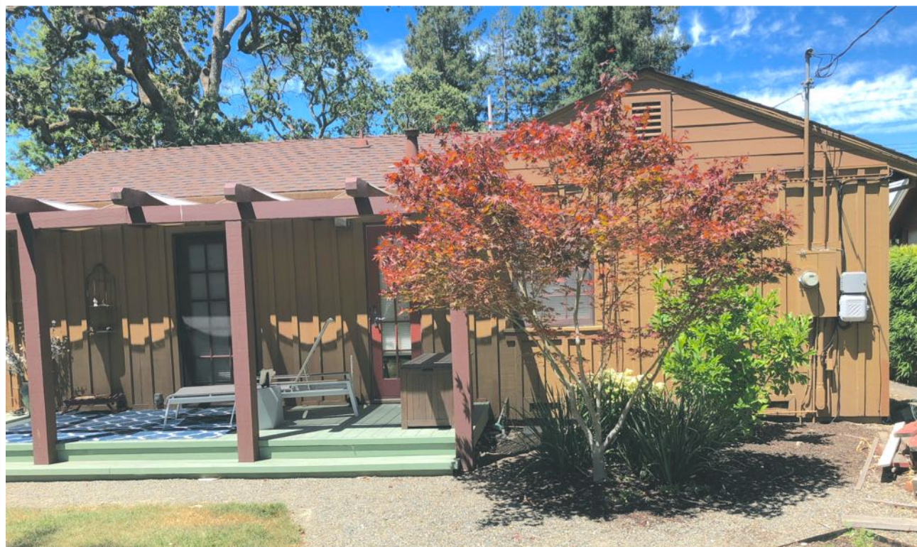
REAR YARD : VIEW LOOKING WEST
