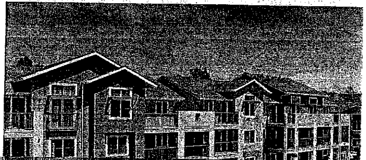
Windsor Redwoods, Windsor Units: 65, Completed: 2011
