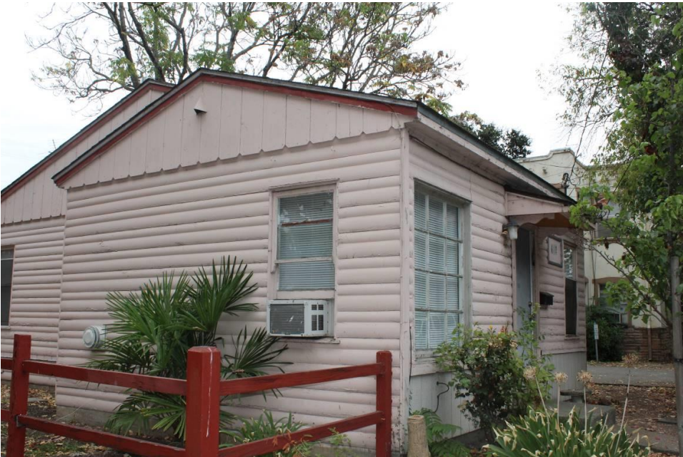
Photograph 4: 612 Morgan Street, northwest and southwest elevations, camera facing east, October 27, 2015.
