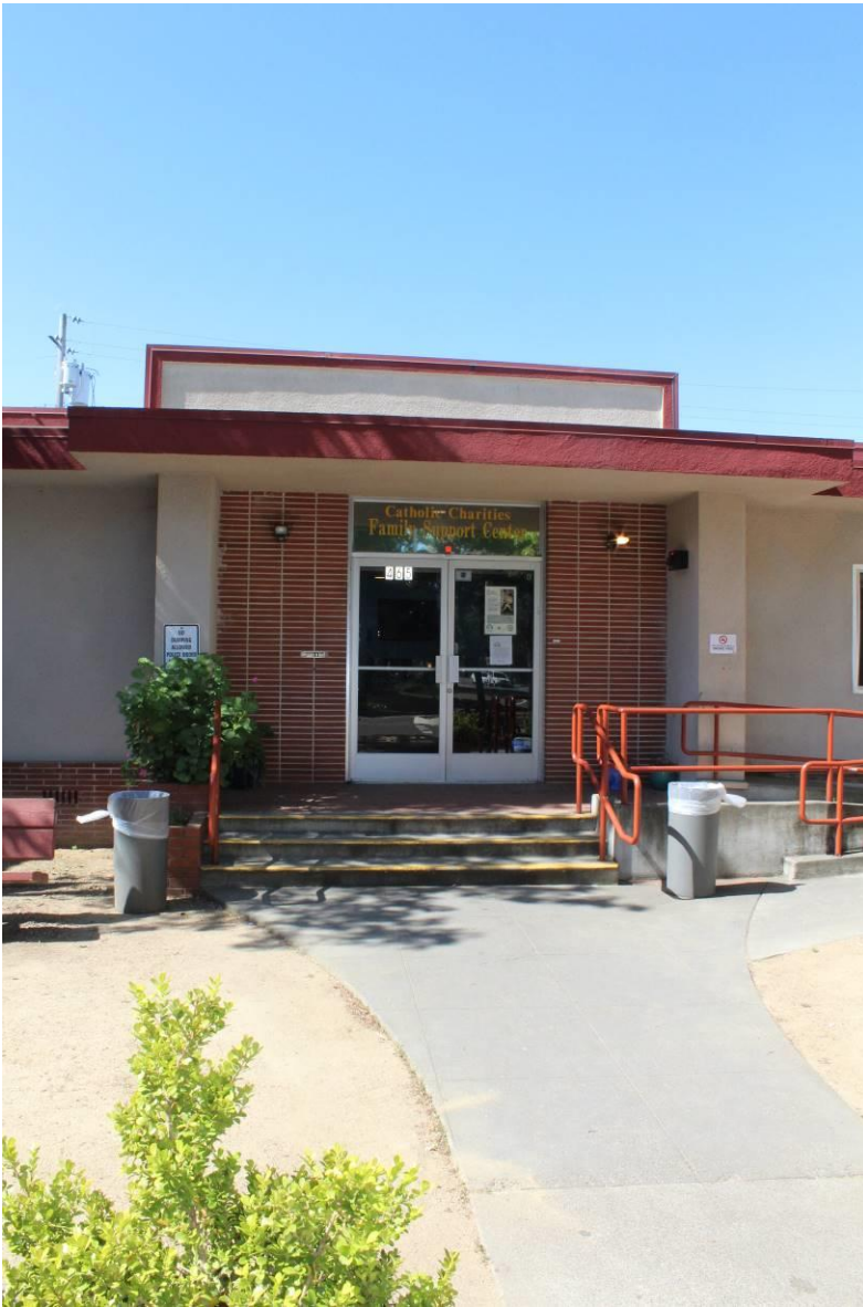
Photograph 4: Detail main entrance, camera facing southwest, April 1, 2016.
