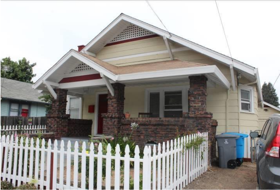
Photograph 8: West elevation, camera facing northeast, August 22, 2018.
