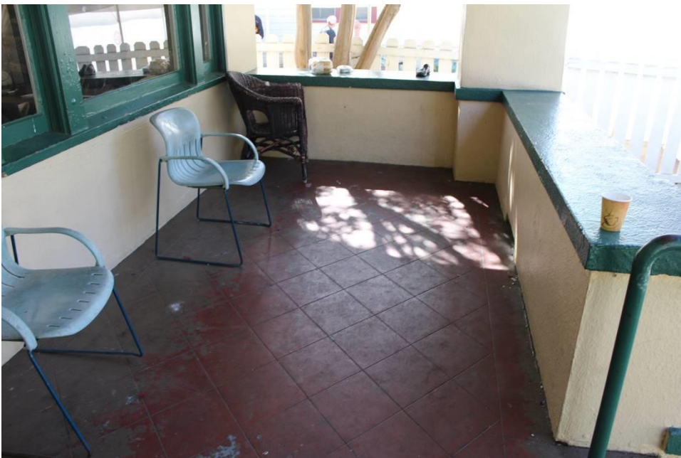
Photograph 5: Detail, front porch, April 1, 2016.
