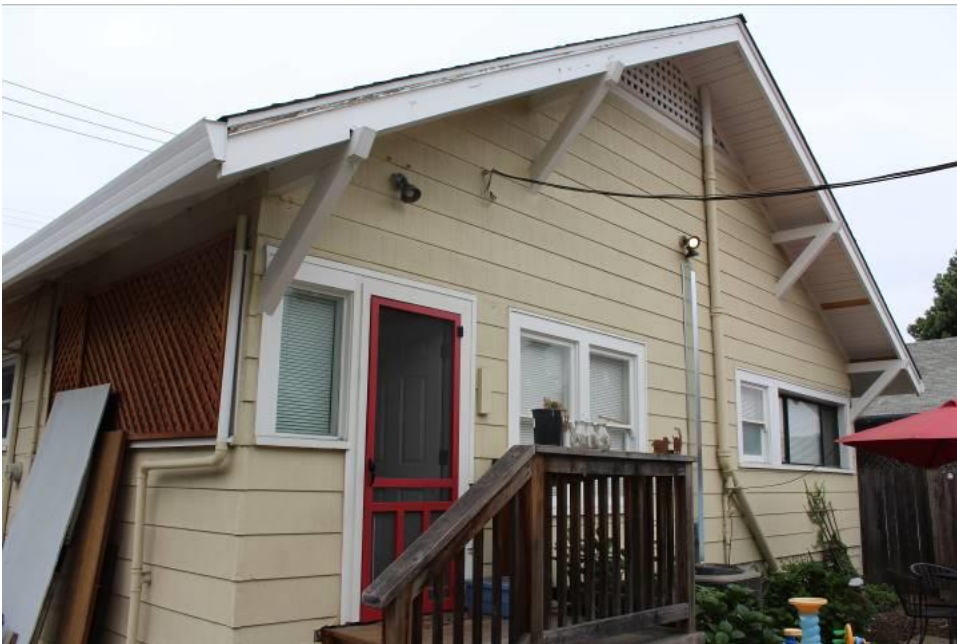
Photograph 5: East elevation, camera facing northwest, August 22, 2018.
