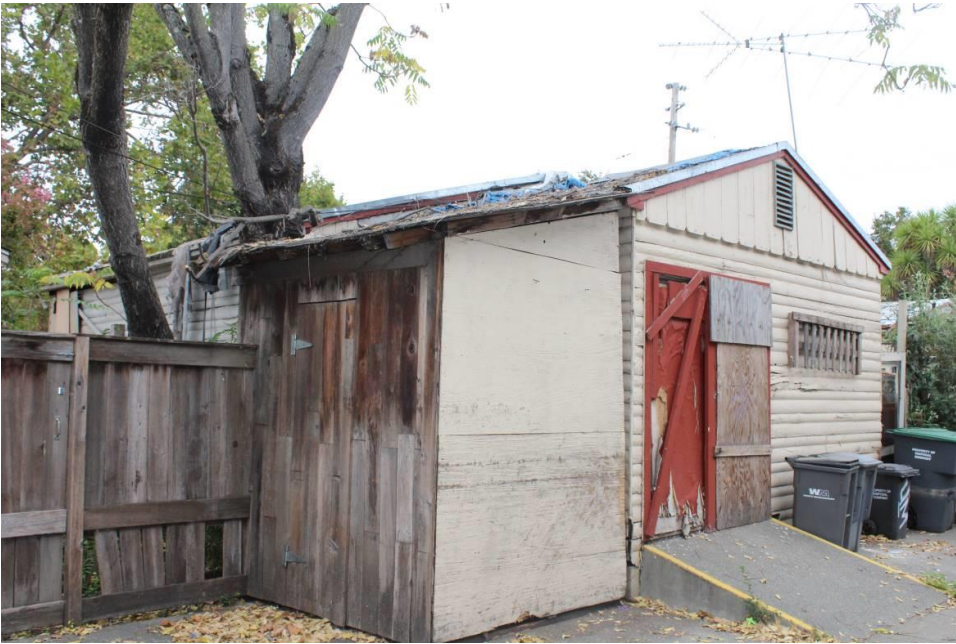
Photograph 9: 304 Seventh Street, southeast and southwest elevations, camera facing northeast, October 27, 2015.
