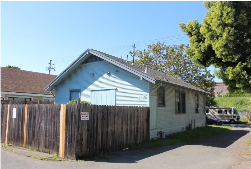
Photograph 4: Northeast and northwest elevations, camera facing south, April 1, 2016.
