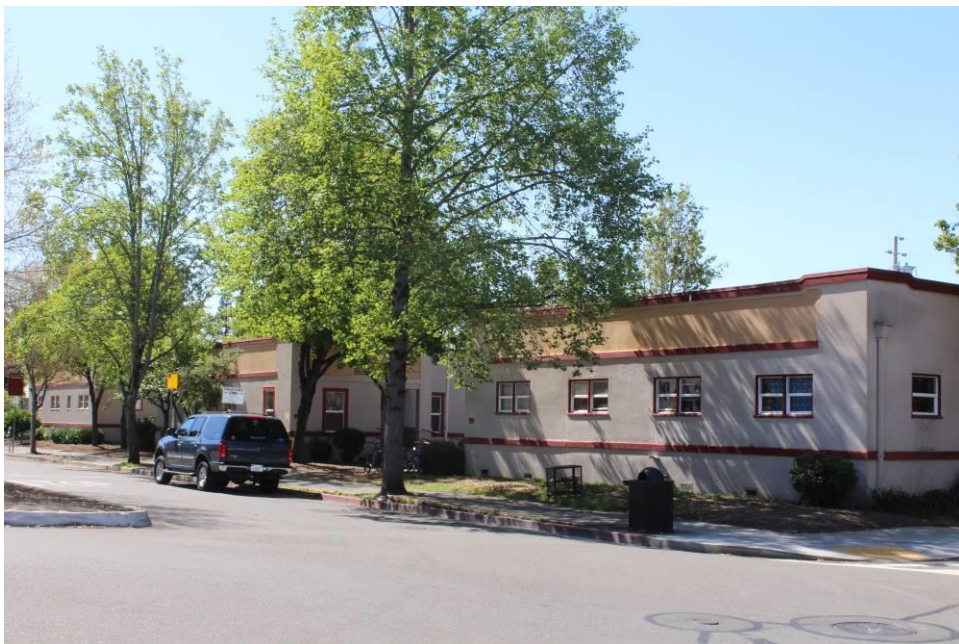
Photograph 2: Northeast and northwest elevations, camera facing south, April 1, 2016.
