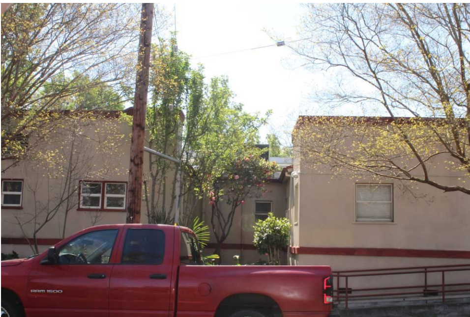
Photograph 8: Northwest elevation, camera facing southeast, April 1, 2016.
