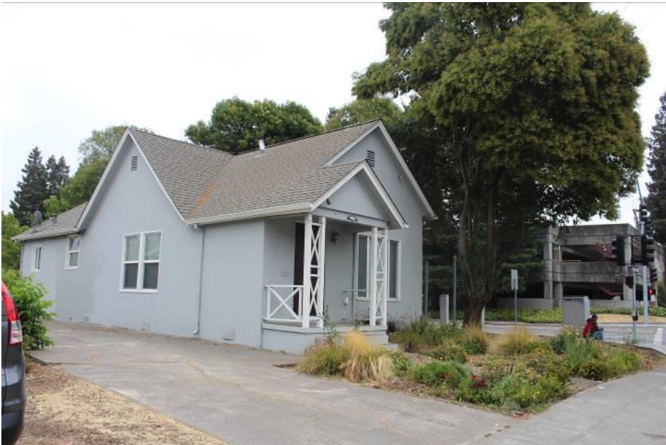
Photograph 3: West and north elevations, camera facing southeast, August 22, 2018.
