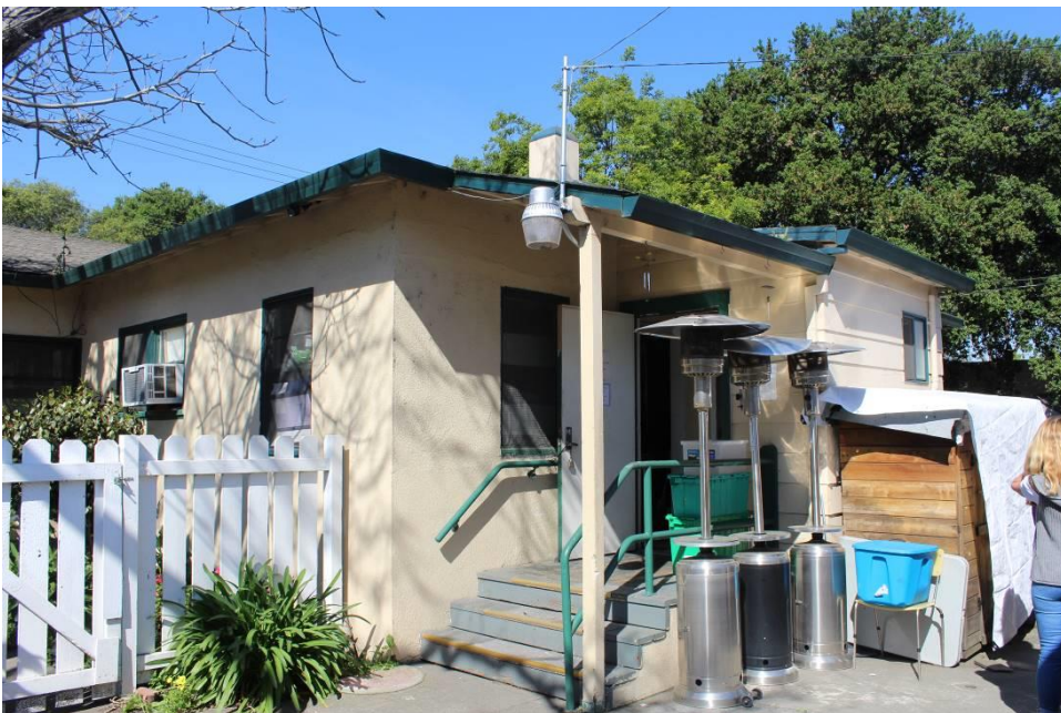
Photograph 3: Southeast and northeast elevations, camera facing west, April 1, 2016.
