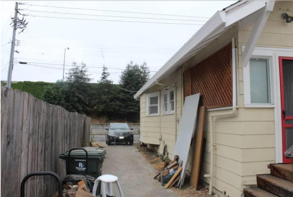
Photograph 6: South elevation, camera facing southwest, August 22, 2018.
