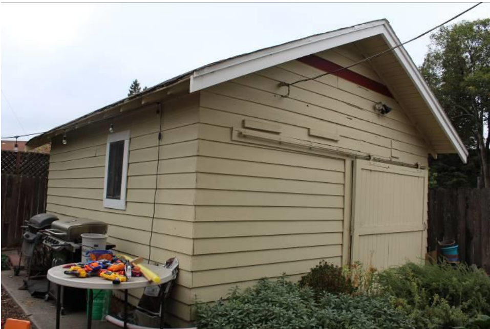
Photograph 9: Garage, north and west elevations, camera facing southeast, August 22, 2018.
