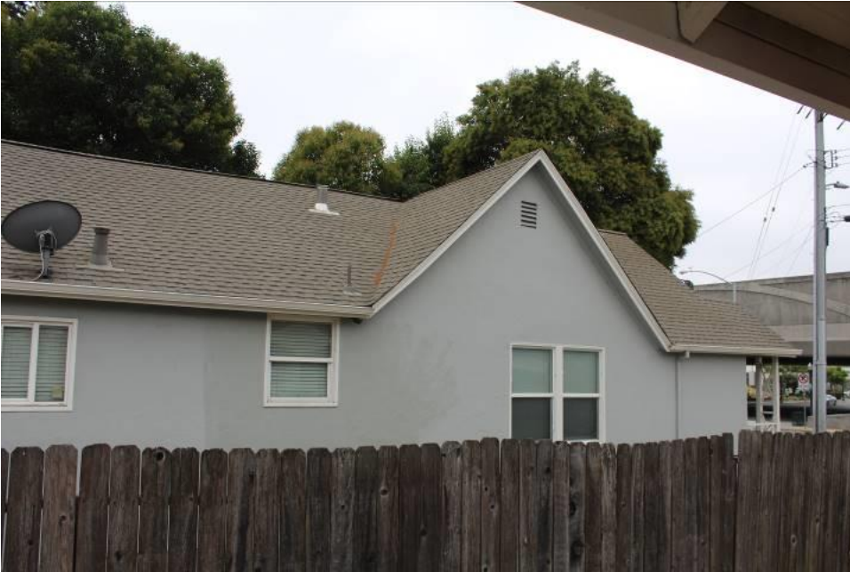
Photograph 4: North elevation, camera facing southwest, August 22, 2018.
