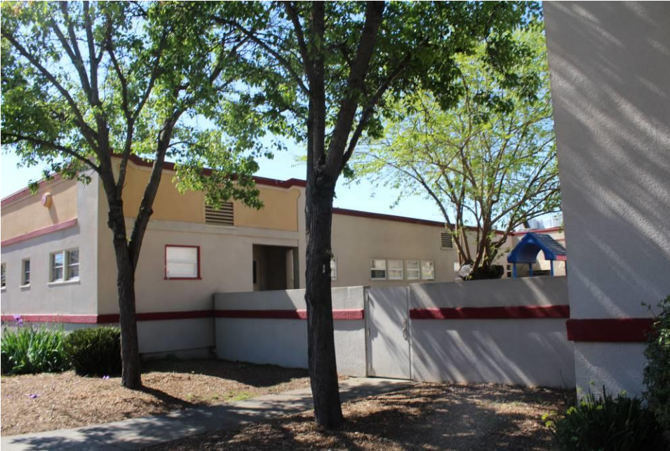
Photograph 5: Northeast and northwest elevations of south wing, camera facing south, April 1, 2016.
