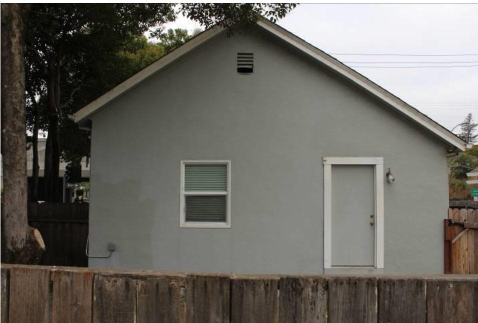
Photograph 5: East elevation, camera facing west, August 22, 2018.
