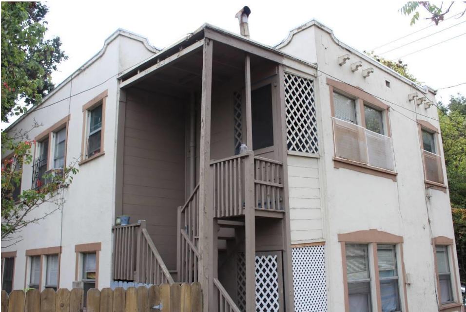
Photograph 4: Northwest and northeast elevations, camera facing south, October 27, 2015.
