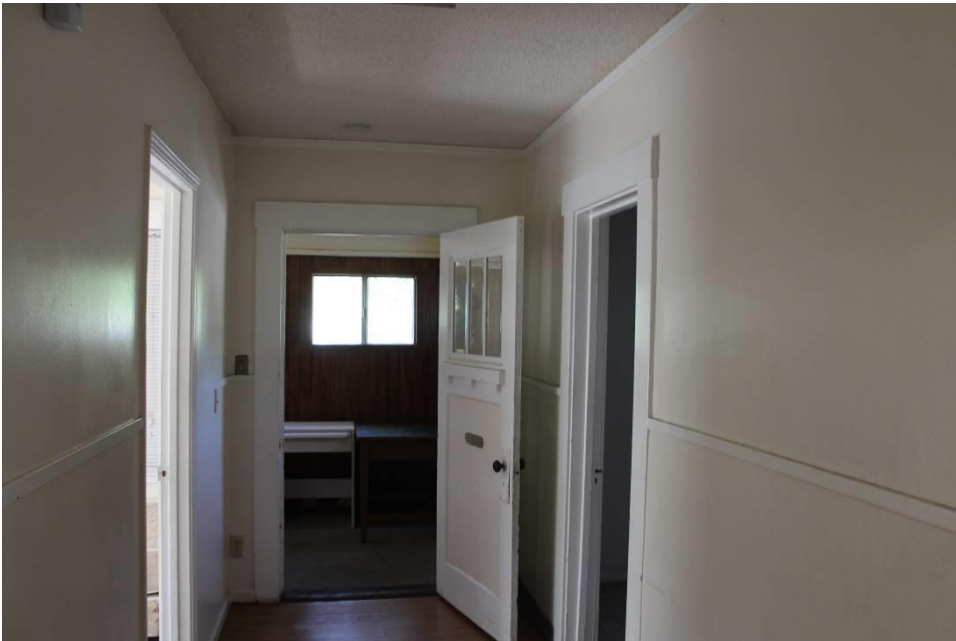
Photograph 7: Interior, hallway, facing into enclosed front porch showing original front door, April 1, 2016.
