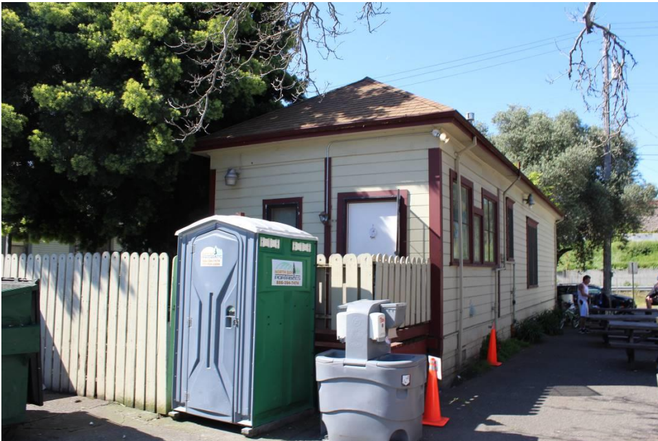
Photograph 5: Northeast and northwest elevations, camera facing south, April 1, 2016.
