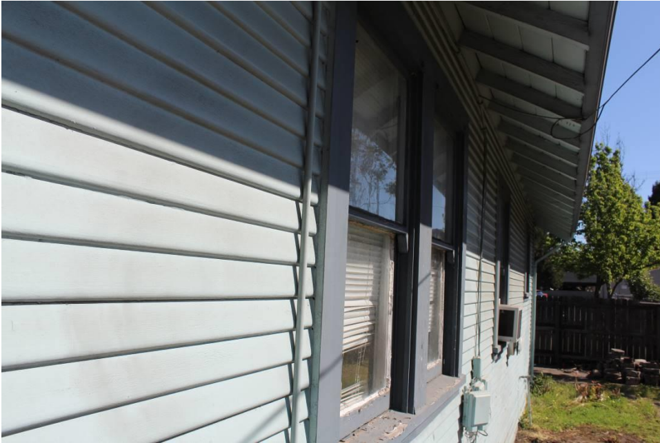
Photograph 2: Detail, southeast elevation, camera facing north, April 1, 2016.
