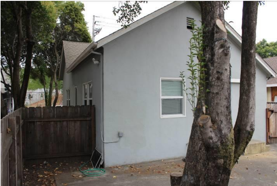
Photograph 6: East and south elevation, camera facing west, August 22.
