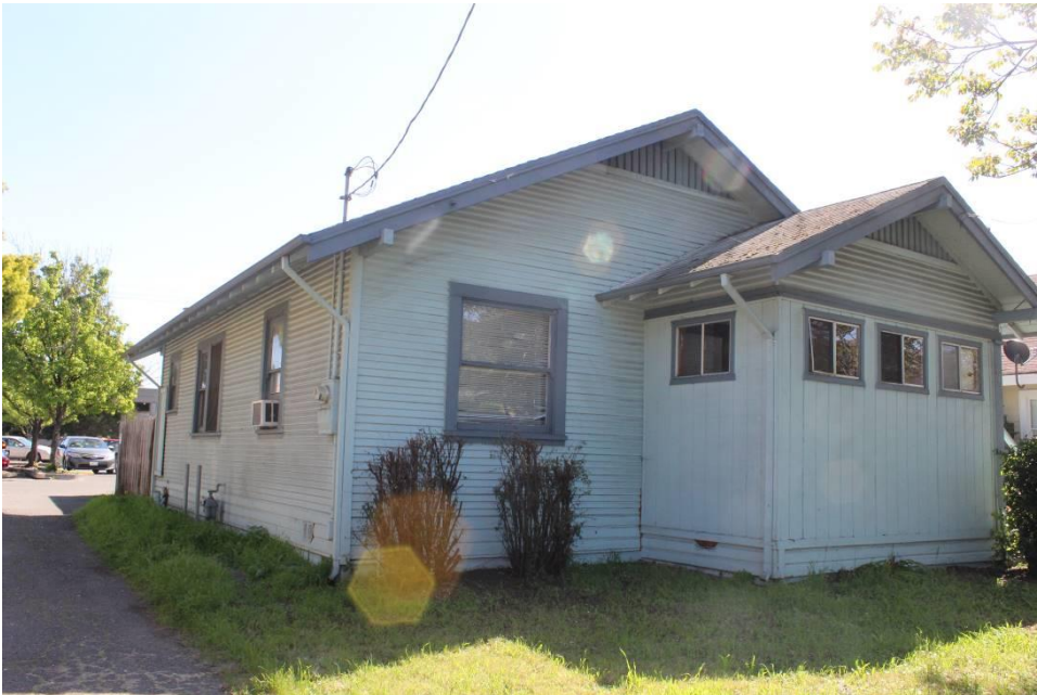
Photograph 5: Northwest and southwest elevations, camera facing east, April 1, 2016.
