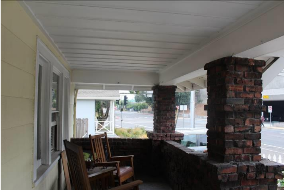
Photograph 2: Detail, west elevation, front porch, camera facing south from porch, August 22, 2018.
