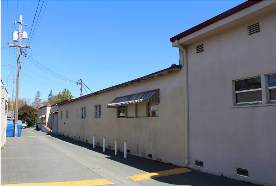
Photograph 7: Southwest elevation, camera facing northeast, April 1, 2016.
