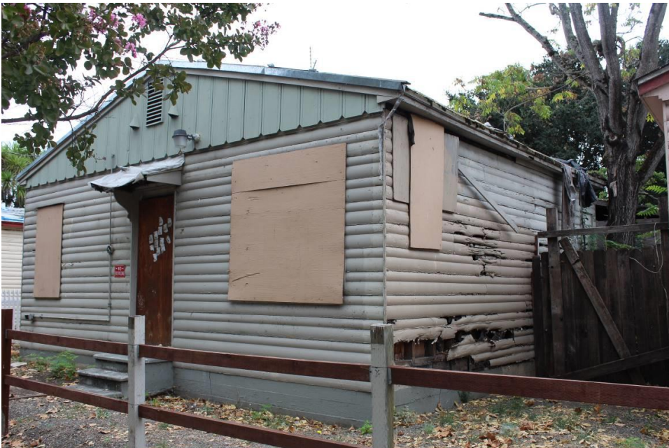
Photograph 6: 304 Seventh Street, northwest (main) and southwest elevations, camera facing southeast, October 27, 2015.
