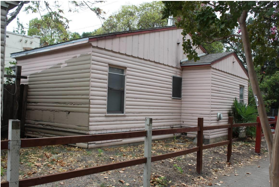
Photograph 5: 612 Morgan Street, northwest and northeast elevations, camera facing southwest, October 27, 2015.
