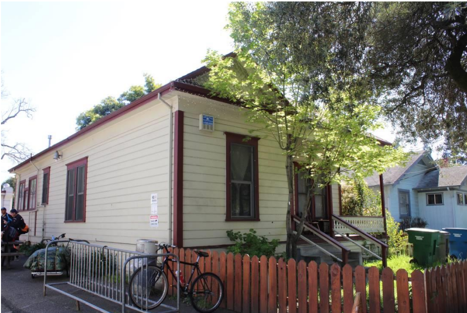
Photograph 7: Northwest and southwest elevations, camera facing east, April 1, 2016.
