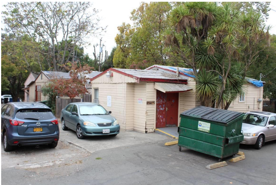
Photograph 2: 306 Seventh Street, northeast and southeast elevations with 304 Seventh Street and 612 Morgan Street showing in background, camera facing northwest, October 27, 2015.
