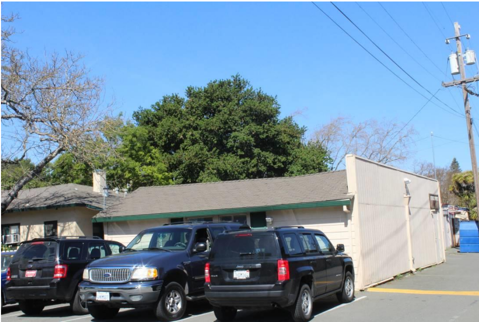
Photograph 8: Rear building, southeast and northeast elevations, camera facing west, April 1, 2016.
