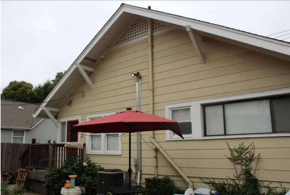
Photograph 4: East elevation, camera facing southwest, August 22, 2018.
