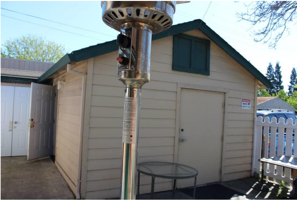
Photograph 6: Rear building, southwest and northwest elevations, camera facing east, April 1, 2016.
