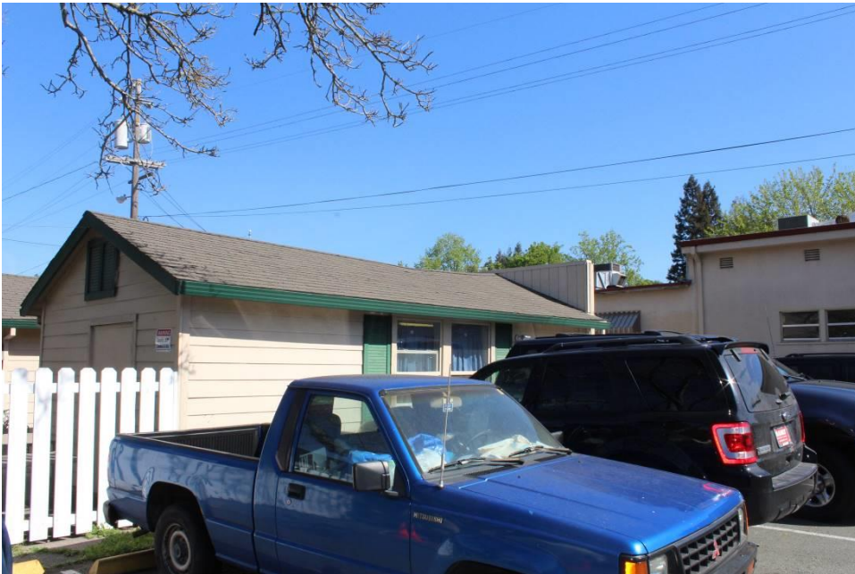
Photograph 7: Rear building, southwest and southeast elevations, camera facing north, April 1, 2016.
