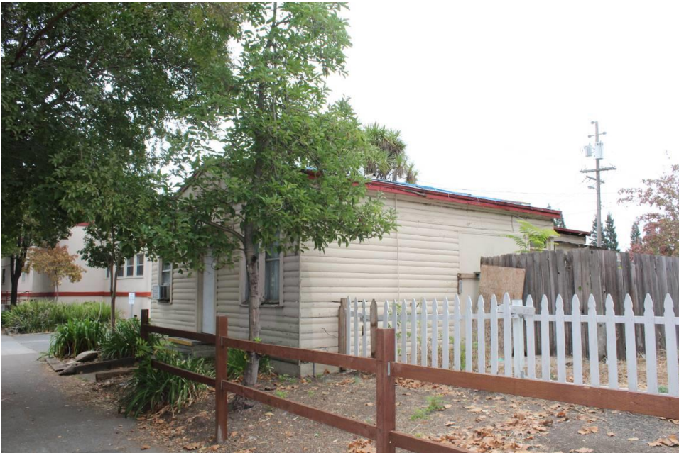
Photograph 12: 306 Seventh Street, northwest and southwest elevations, camera facing east, October 27, 2015.
