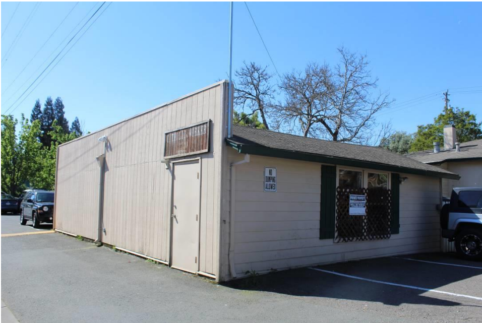
Photograph 9: Rear building, northeast and northwest elevations, camera facing south, April 1, 2016.
