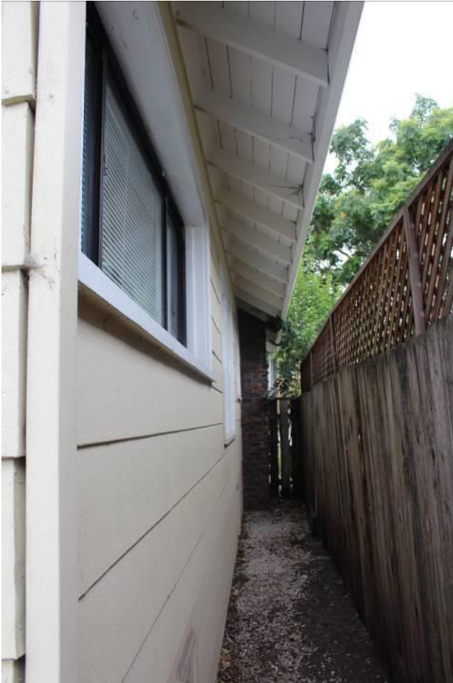
Photograph 3: North elevation, camera facing southwest, August 22, 2018.
