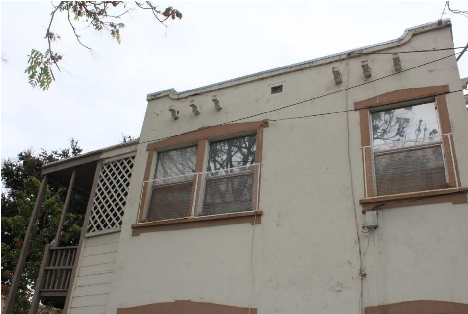
Photograph 3: Second story, northwest elevation, camera facing southwest, October 27, 2015.
