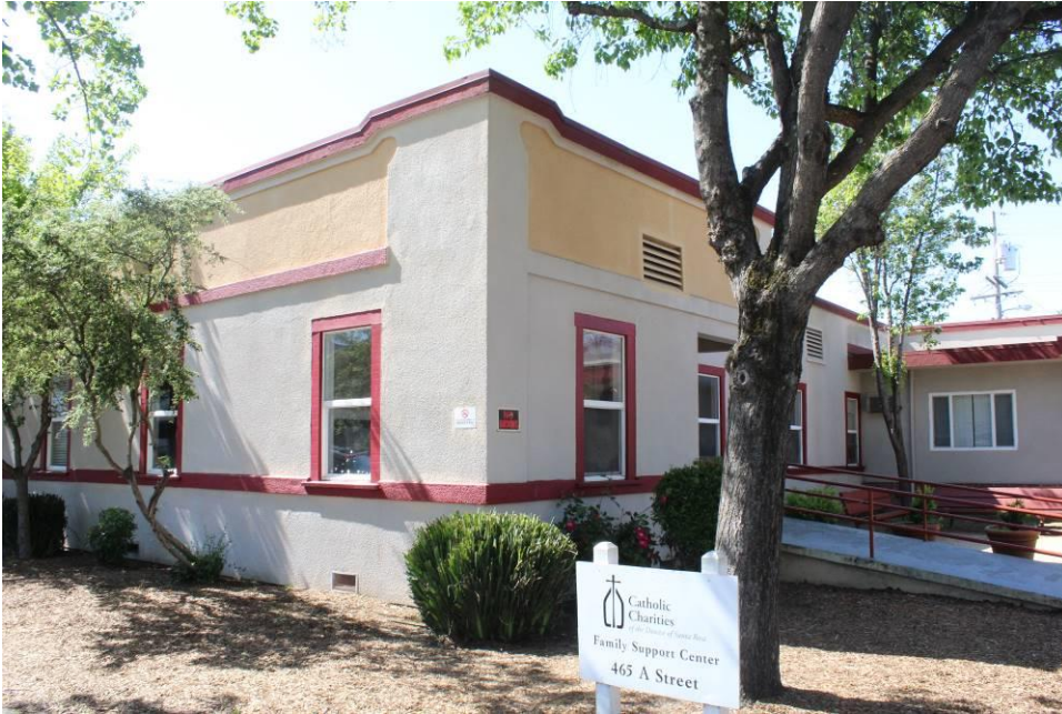
Photograph 3: Northeast and northwest elevations of center wing, camera facing south, April 1, 2016.
