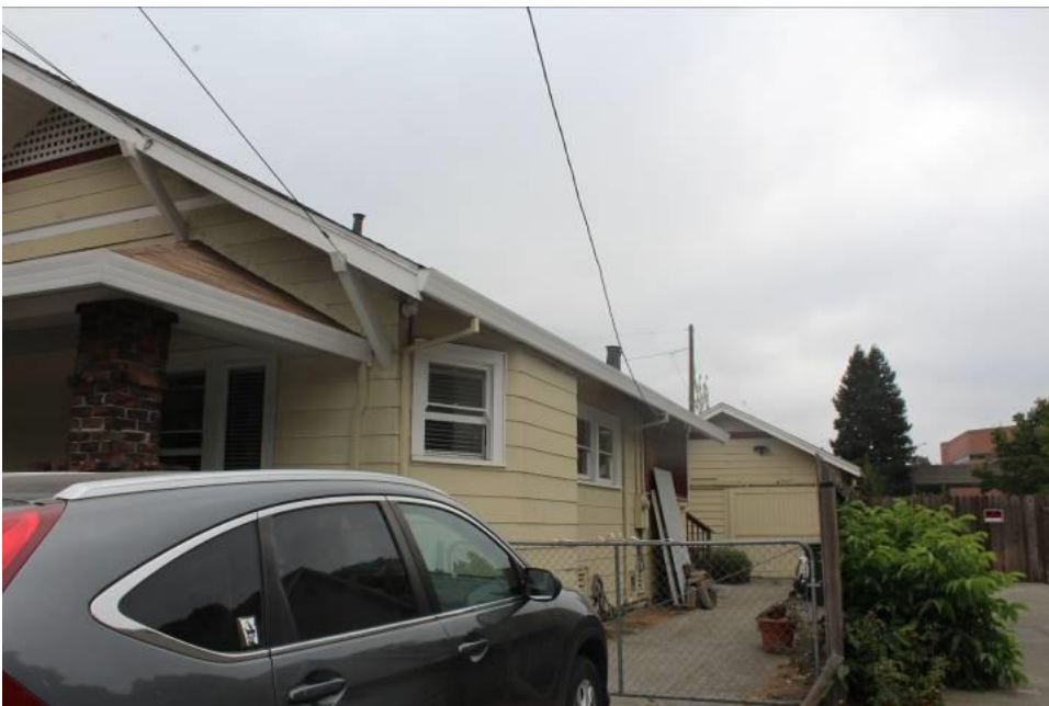
Photograph 7: South elevation, camera facing northeast, August 22, 2018.
