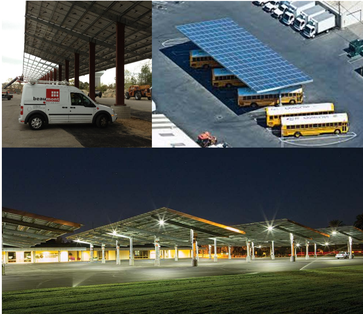
Figure 7-3: Example Solar PV Carport Structures
