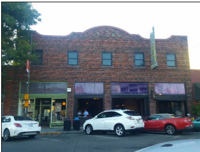
Jacobs Building south façade, 111-115 Fourth Street
