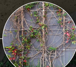
Wire Rope Trellis System
