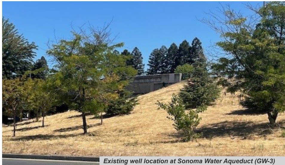
Existing well location at Sonoma Water Aqueduct (GW-3)
