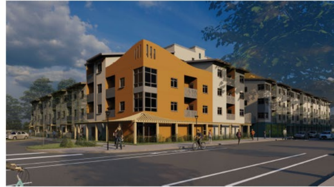
MAIN BUILDING CORNER
