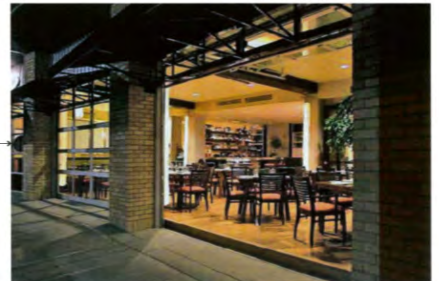
ROLL-UP DOORS AT RESTAURANT
