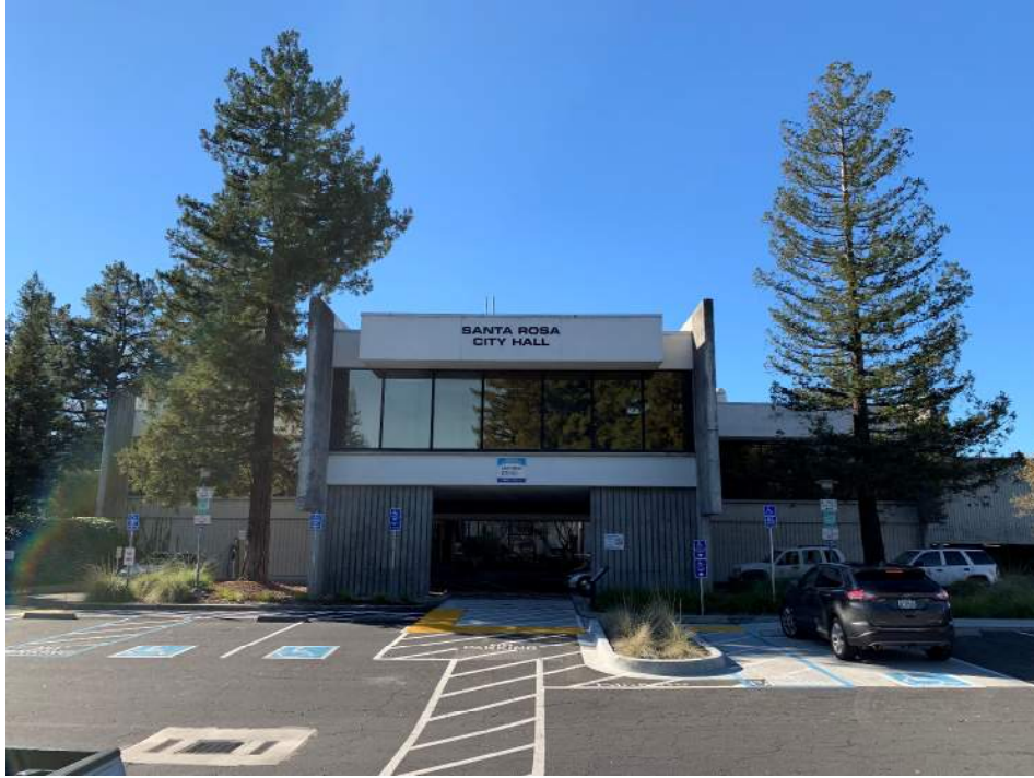
Figure 9: Building 8 (Right), Building 9 (Center) and Building 10 (Left) Elevation
