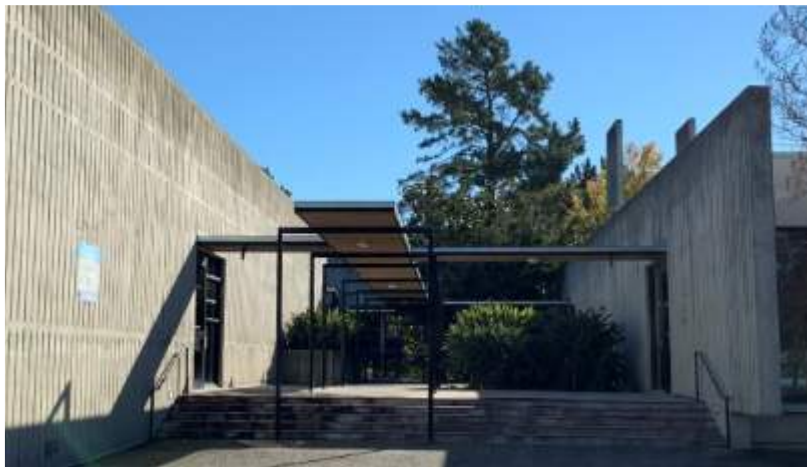
Figure 12: Entry Canopy Between Building 5 and 6
