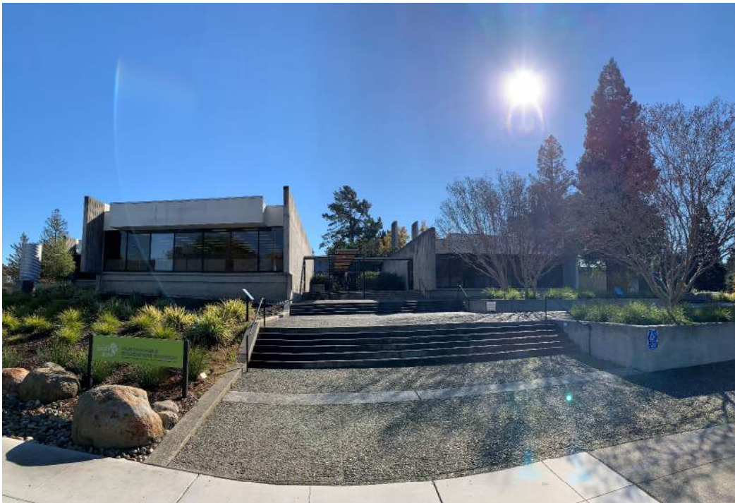
Figure 8: Building 5 (Right) and Building 6 (Left) Elevation. Building 7 to the Left of Building 6
