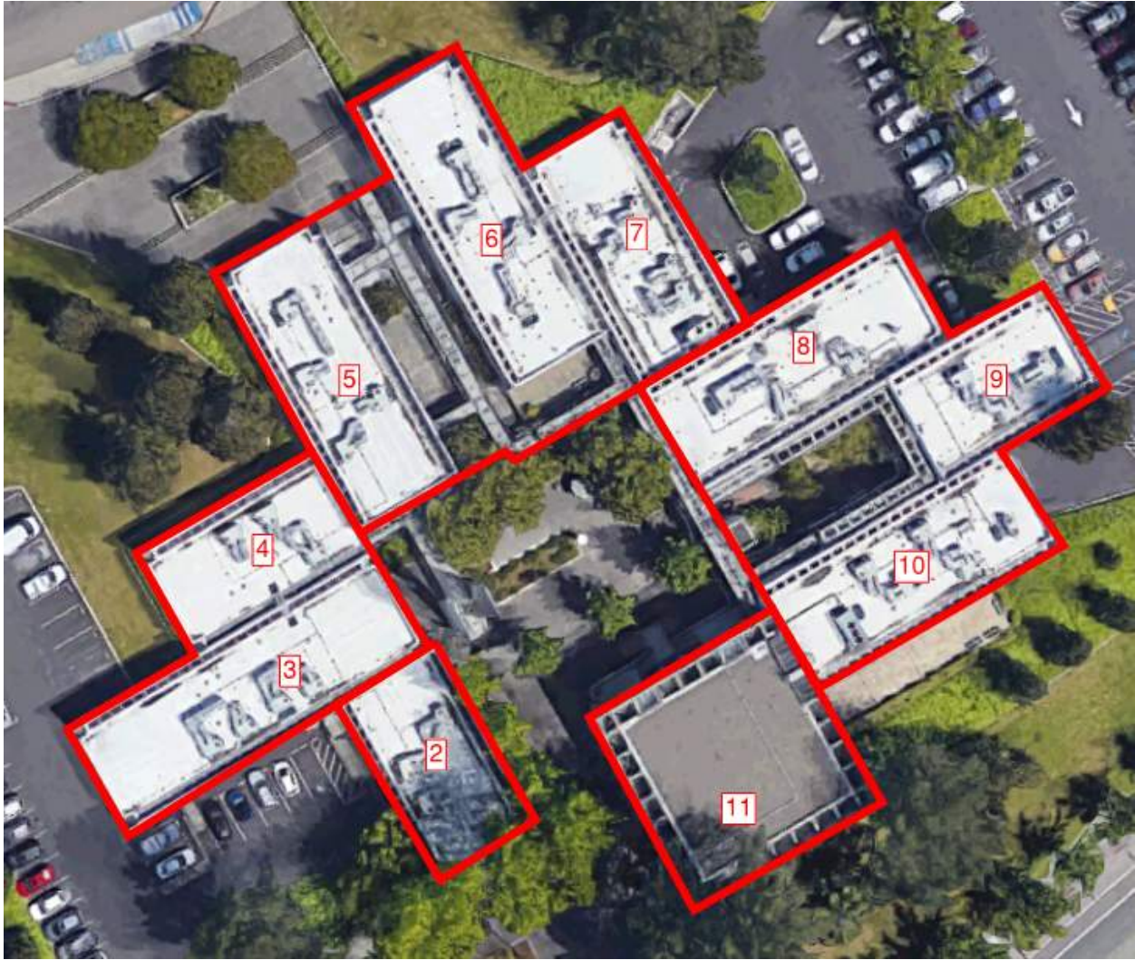
Figure 3: Santa Rosa City Hall - Aerial View
