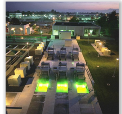
Laguna Treatment Plant
