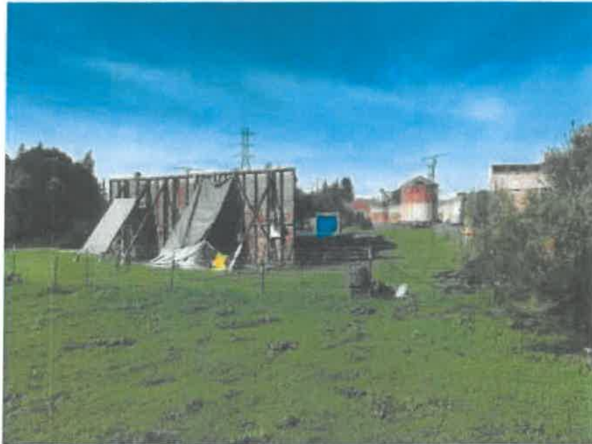
View of the project site from looking north.
