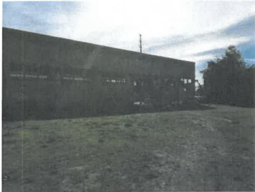
View of the project site from looking southeast.
