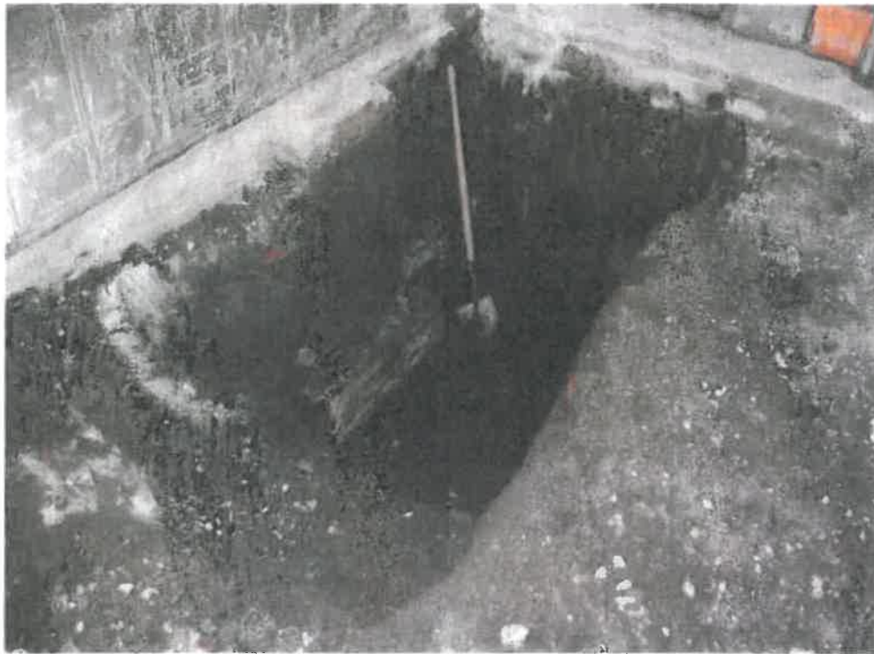
Interior footing on east side of building.
