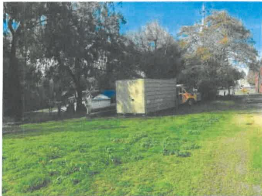
View of materials within project site.
