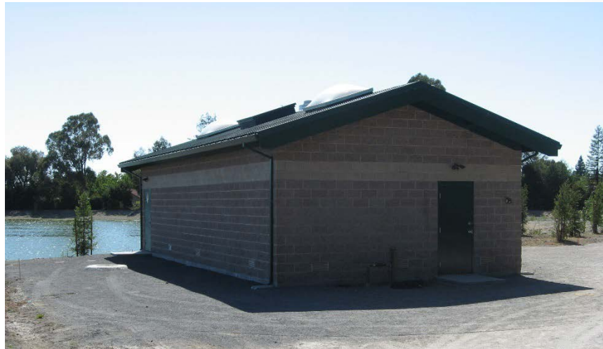
Existing Recycled Water Pump Station installed in 2008
