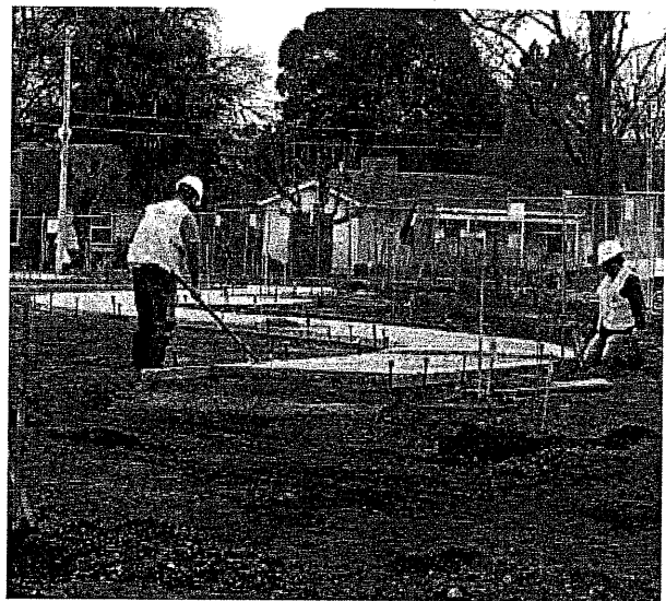
Pathway construction at Finali Park
