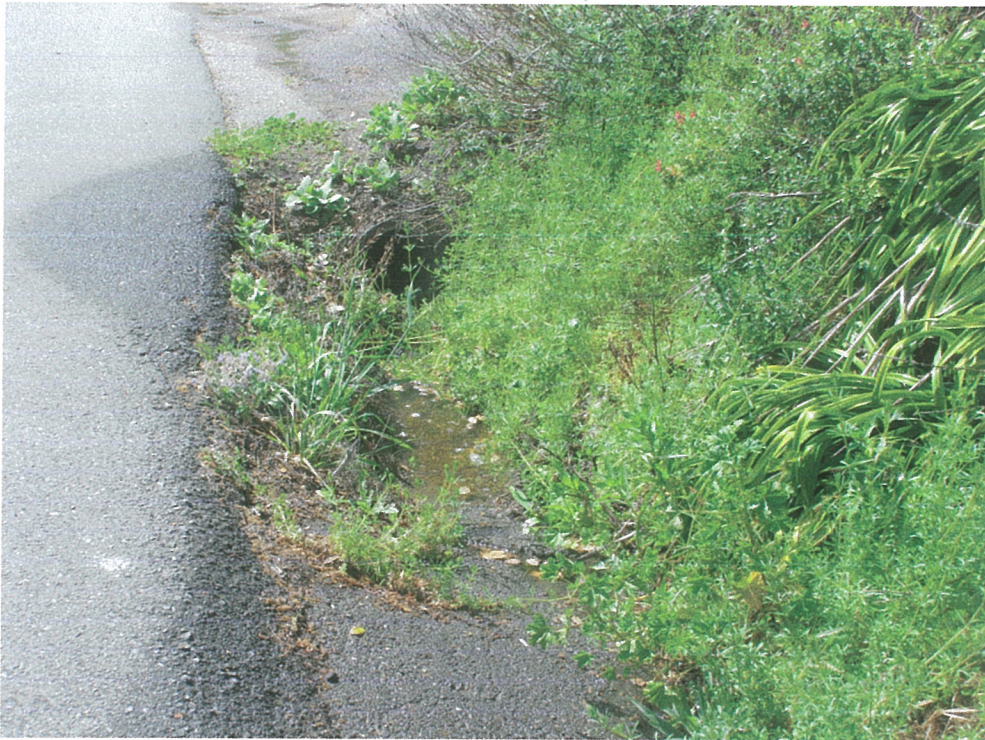
Figure 7. Storm drains would be extended by 27' within the existing ditch on the north side of Chanate Road.
