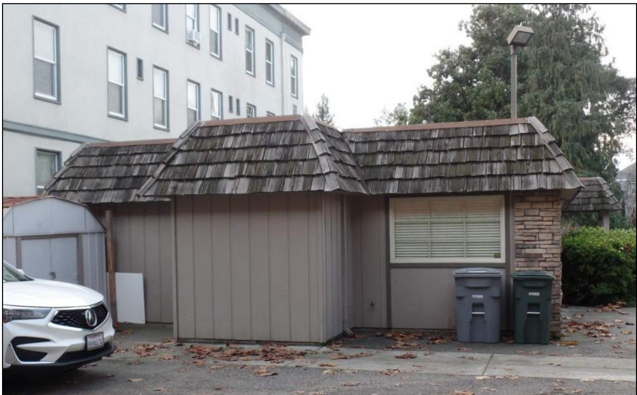
528 B Street east façade, view to west
