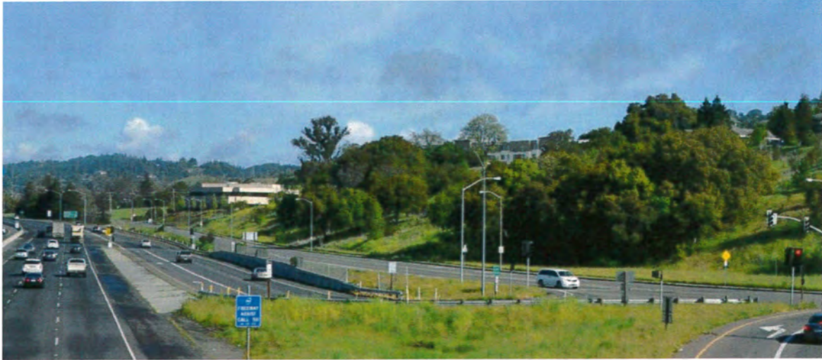
View 3. Looking at building site north from overpass on 101. Only upper levels of the proposed building are visible between the existing tree groves.
