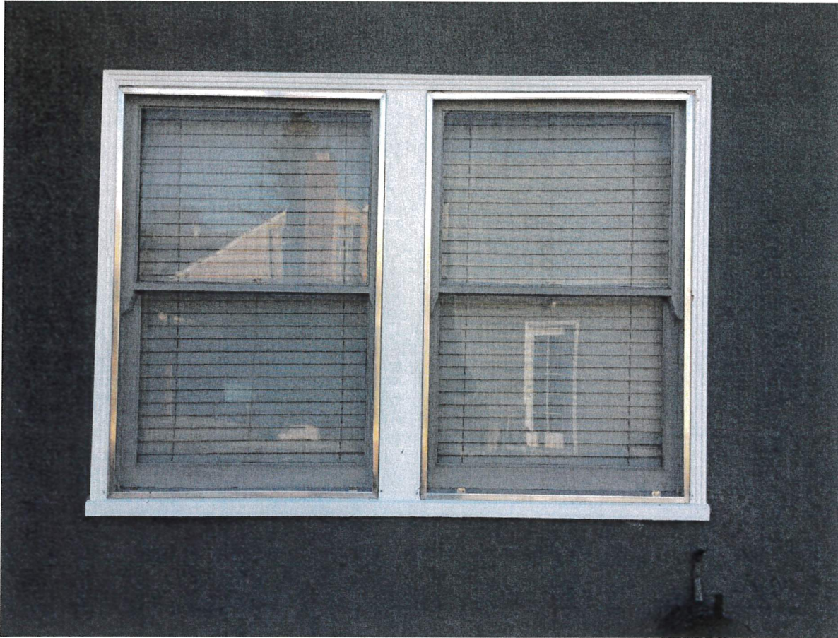
Windows 5 and 6 – Bedroom windows
