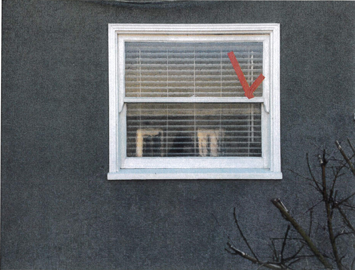
Window 4 – Bathroom window
