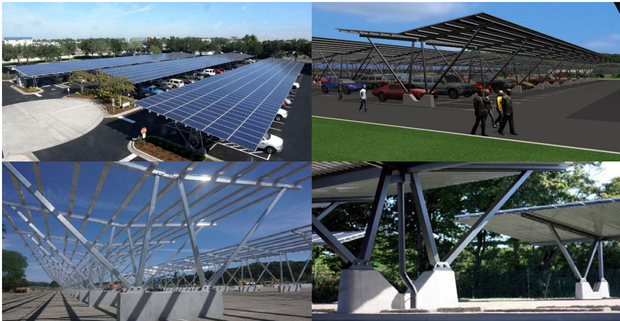
Figure 7-2: Example Solar PV Carport Structures
