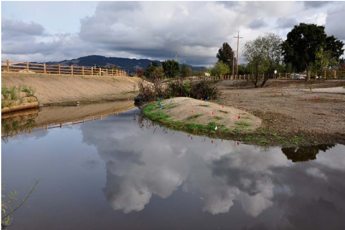
Restoration of Colgan Creek
