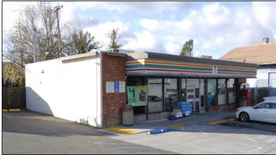
Figure 7: Existing convenience market built in 1968.
