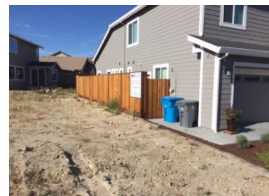
Figure 4 Wooden Fence Attached to Structure
