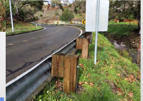
101 Metal beam burned guardrail posts replaced
