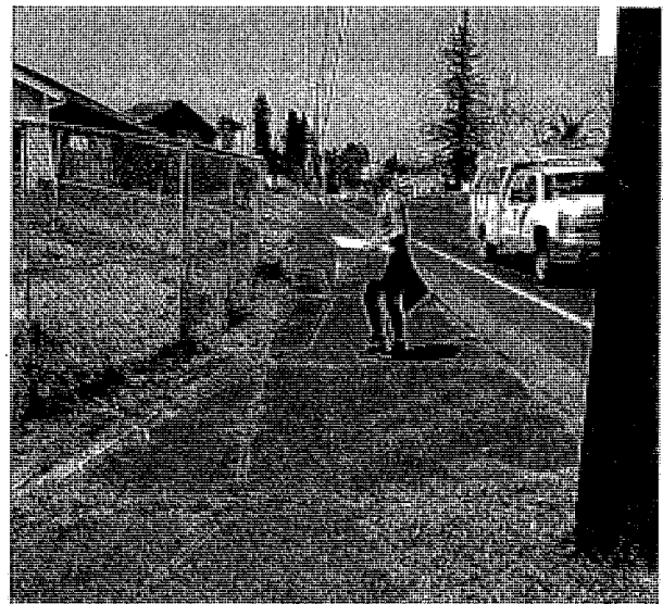
Carlile Macy staff confirming existing site conditions in Coffey Park
