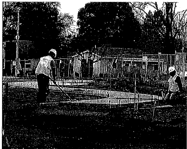
Pathway construction at Final Park
