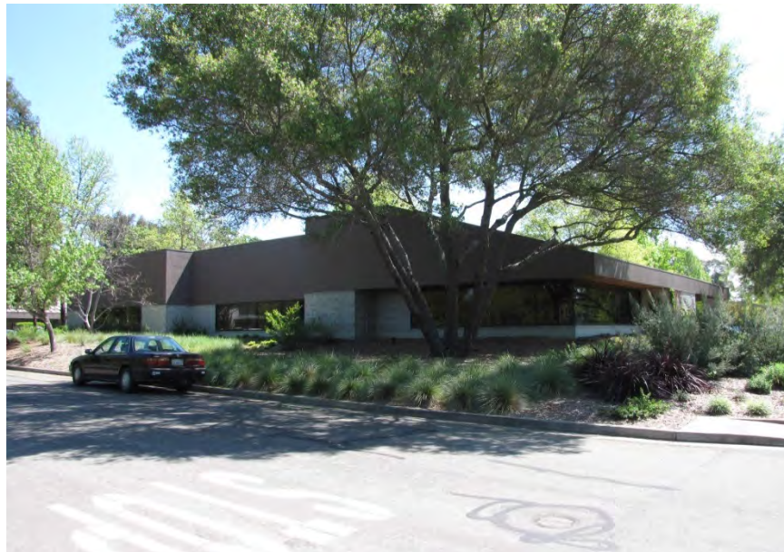
Figure 12: Office park southwest of the Jennings Avenue crossing site.
