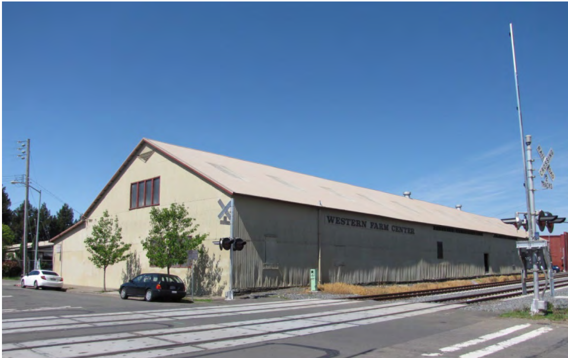
View 3: View of the American Produce Company warehouse at the W. Seventh Street crossing looking northwest.
