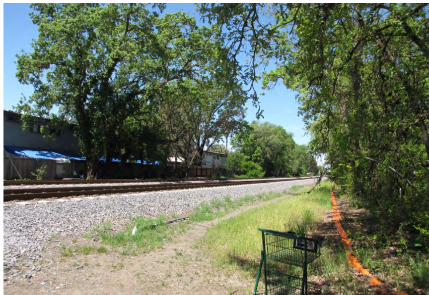
Figure 10: Railroad tracks at Jennings Avenue looking northwest.
