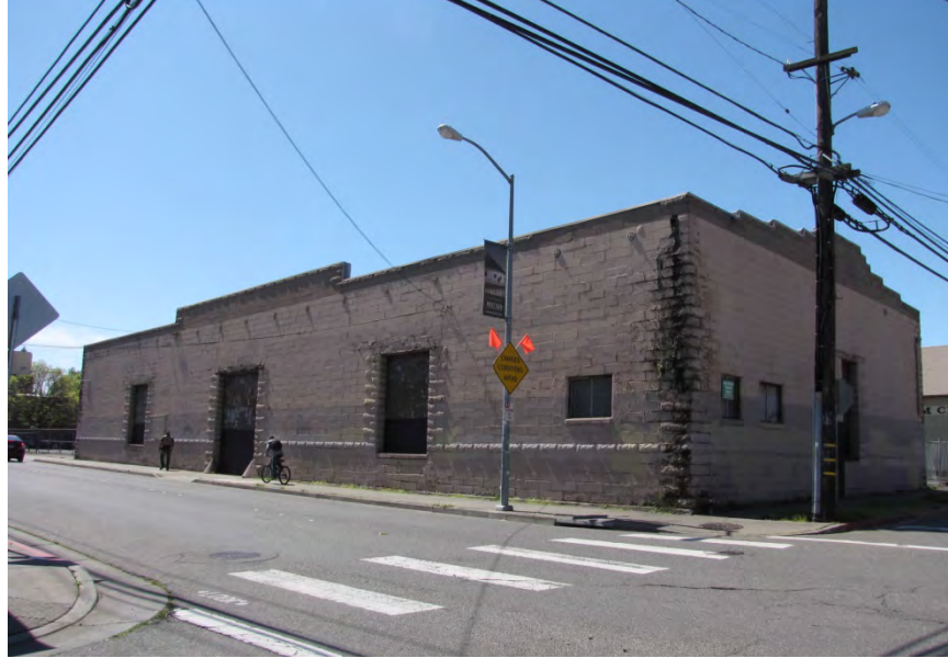
Figure 25: View of the Lee Brothers & Company warehouse at West Eighth and Wilson Street looking southwest.
