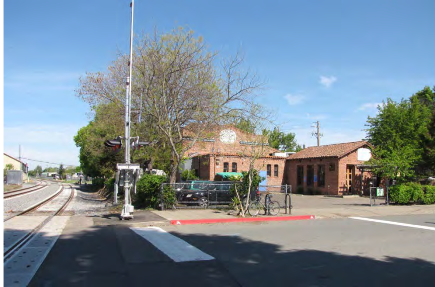
Figure 19: View of the Santa Rosa Flour Mill at the West Sixth Street crossing looking north.
