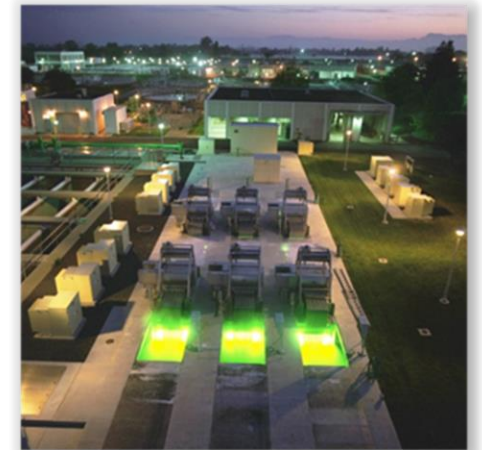
Laguna Treatment Plant
