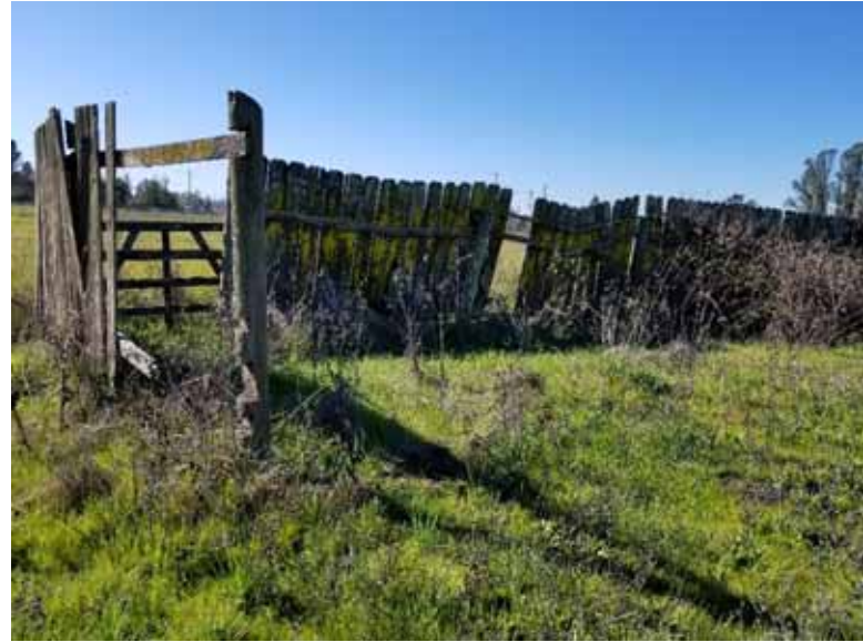
Fence On Northern Portion of Property
