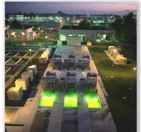
Laguna Treatment Plant
