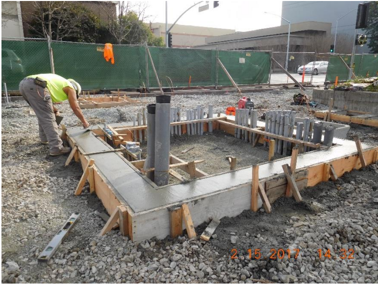
Eastern kiosk foundation
