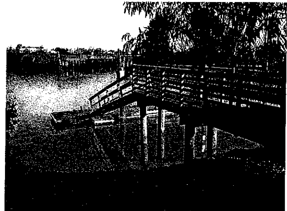
View of Dock on East End of Site
