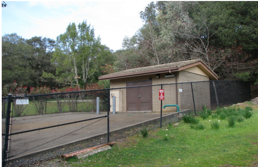
Image 2: View of Existing Emergency Well Facility
