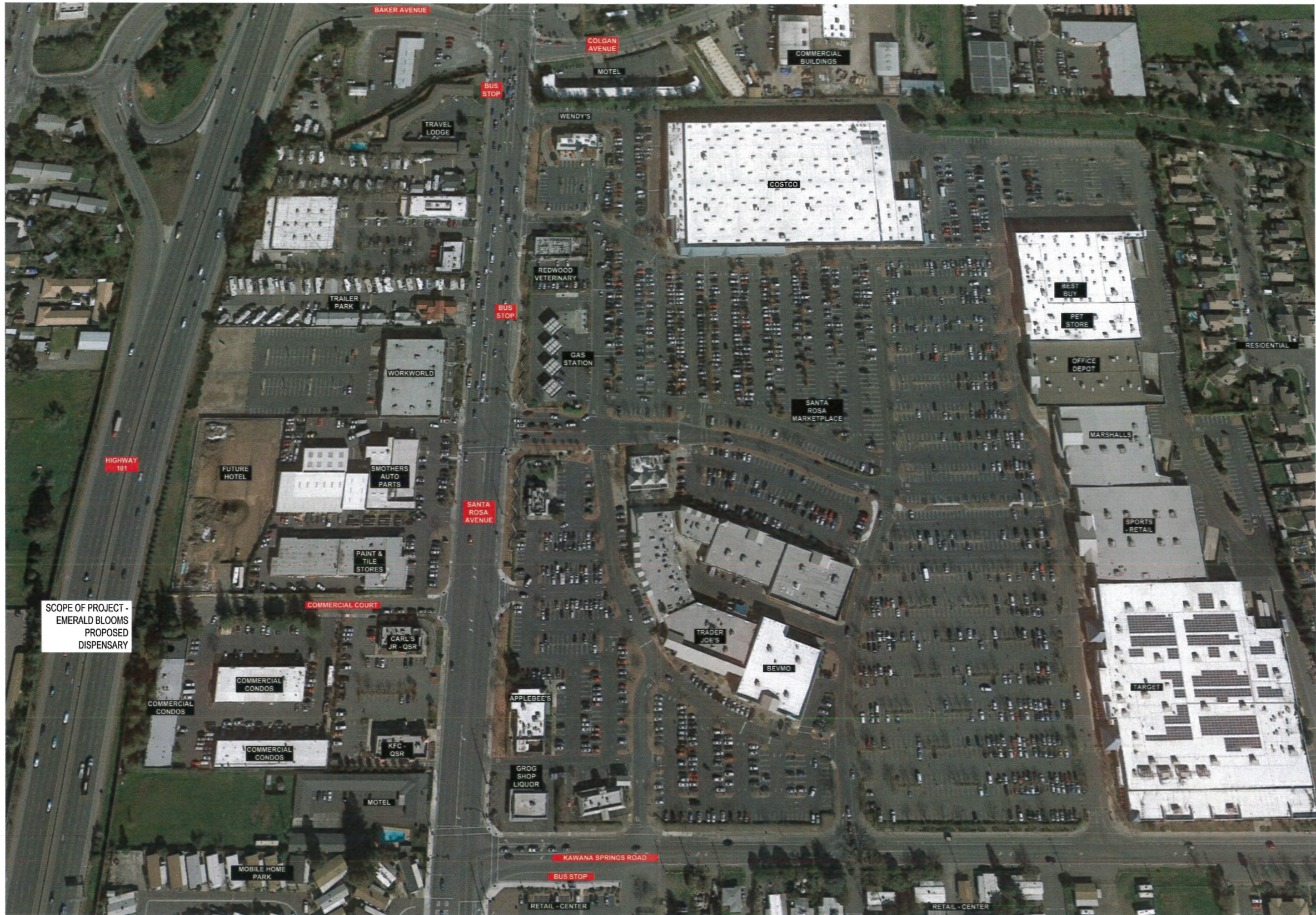
1 AERIAL CONTEXT PHOTO A1.0 1" = 60'
