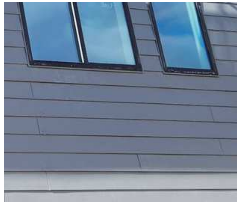
D. FIBER CEMENT BOARD
