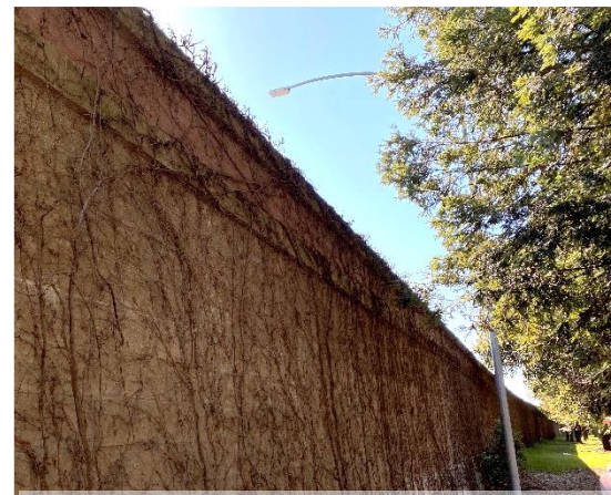
Masonry block wall
