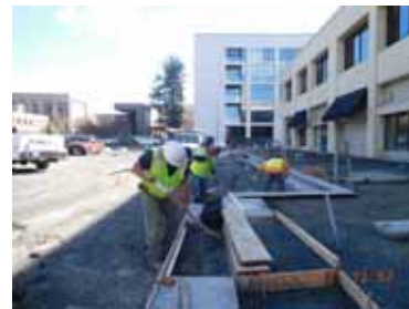
Western sidewalk prep
