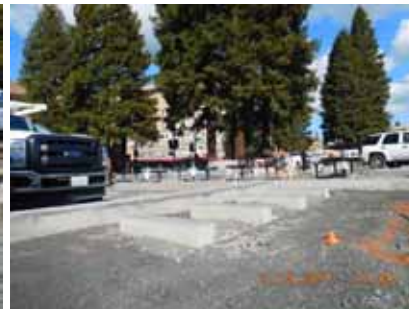
Bike rack foundations
