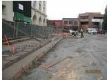
Western roadway prep
